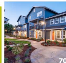
Hayden Bridge Landing 70
